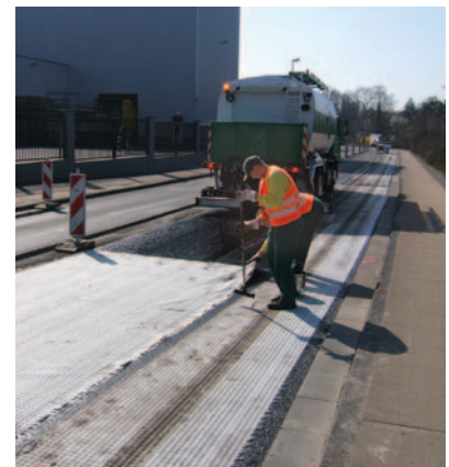
A simple overlap joint for Tensar Glasstex.
