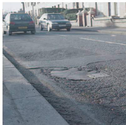
Common structural pavement problems, rutting, fatigue and reflective cracking.
