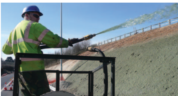
Application of HydraMax erosion control on the M25 Motorway, UK.
