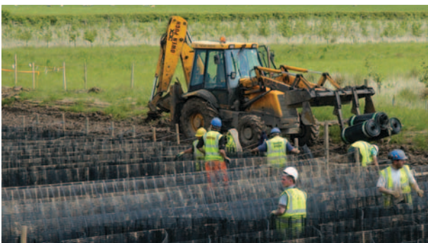
TensarTech® Stratum Foundation Mattress System is used here to control differential settlement over variable ground.
