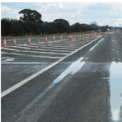
Common structural pavement problems, rutting, fatigue and reflective cracking.
