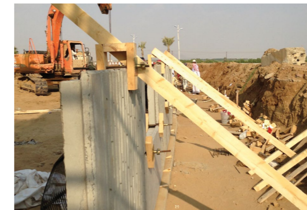
Ares Wall Systems typically require propping on the first course of panels only to ensure correct installation occurs from foundation level.
