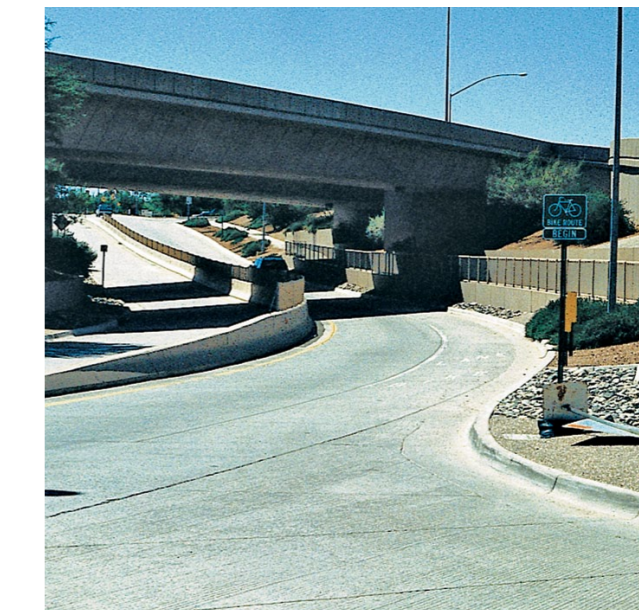
Tanque Verde Interchange, Tucson, Arizona - Constructed in 1984-85, this was one of the first Tensar Walls ever built. This demonstrates the long-term performance of the TensarTech Ares Wall System.
