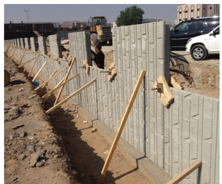
Architectural finishes are easily achieved by the use of rubber liners during panel casting.
