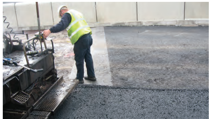
Glasstex®Patch™ 880 can be overlaid by either hand or machine lay operations.
