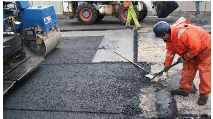
Glasstex®Patch™ 880 can be installed either between the base and binder course or the binder and surface course.
