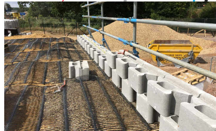
Grafham Road Bridge and B1514 Junction
