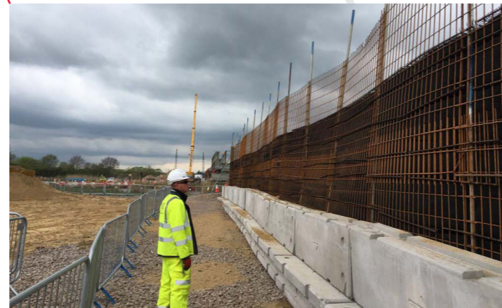
River Great Ouse Viaduct
