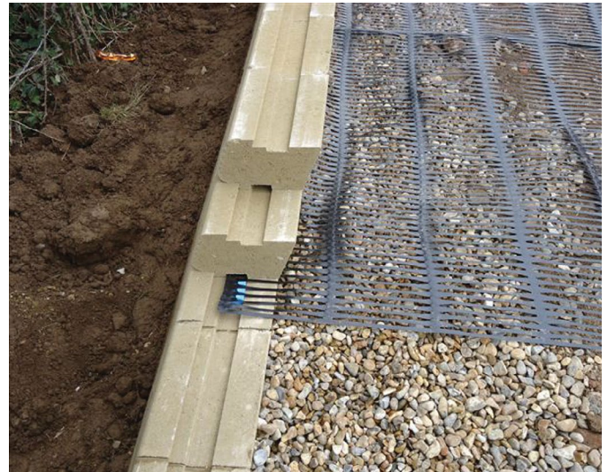
Positive high efficiency connection between TensarTech® SlopeLoc™ facing and Tensar geogrid.
