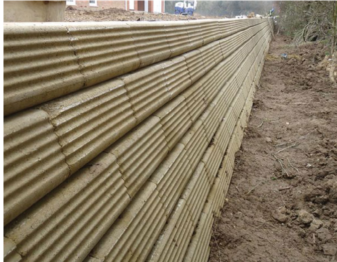
Mortar free construction of modular facing, rapidly installed.
